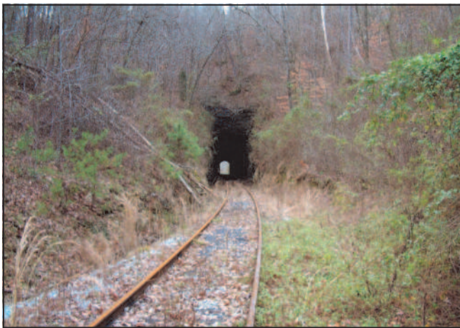
This is the west portal of the tunnel near Flat Top. This end has no mantle dressing the opening. Apparently, the rock at the west end of the tunnel has been stable enough to not require a liner or face support.
