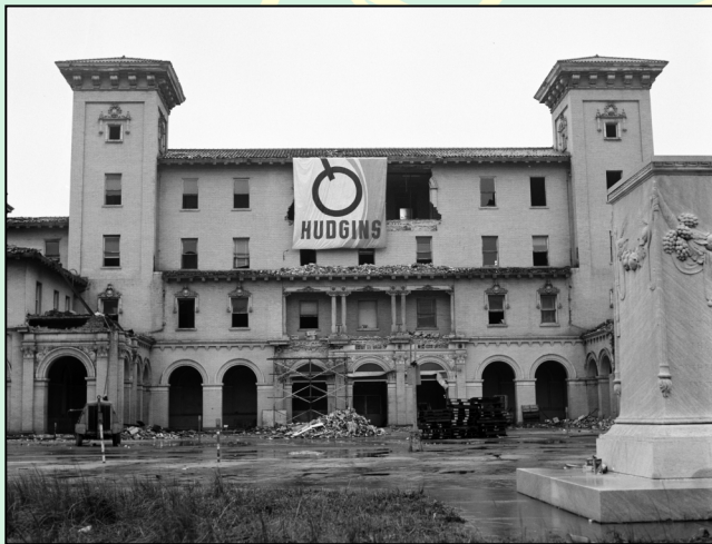
The demolition of Atlanta Terminal Station begins in earnest in 1972. Note how the statue of Samuel Spencer has been removed from its pedestal. It was on display at Peachtree Station, on a small brick pedestal, for 24 years. (Martin K. O'Toole photo)
