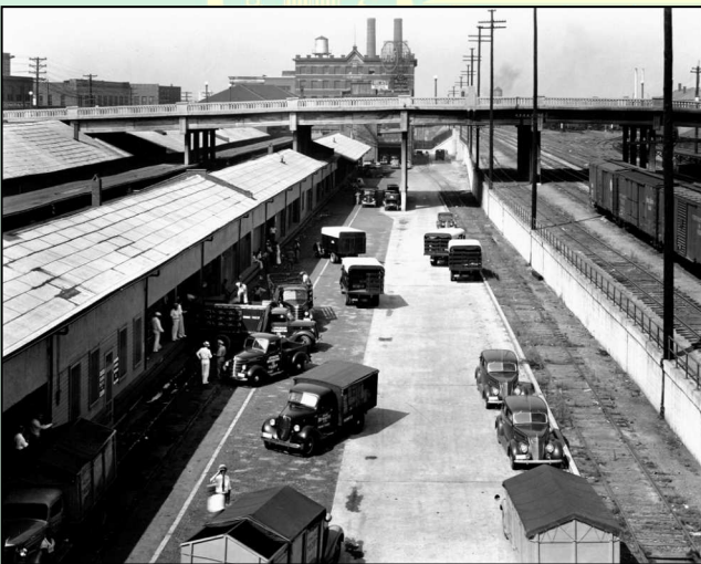
The Southern Railway warehouse/freight house on the south side of the grade separation at the 21 st Viaduct as it appeared in the 1940s. The retaining wall was part of the elevation project as completed in 1933. The “street” was originally an AGS RR right of way. (Birmingham Public Library Collection)
