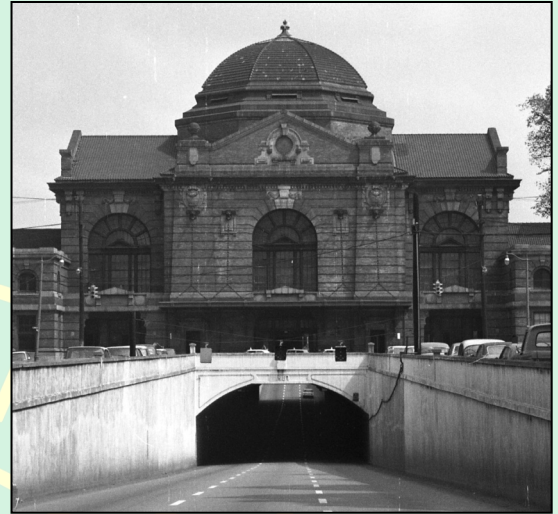
Flooding in the 5th Avenue underpass at Terminal Station led to assurances that the new underpasses for the elevation project would be built with adequate drainage. (Don Phillips photo)
