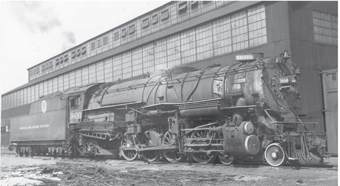
No. 1600 was one of the monstrous 3-cylinder 4-8-2s which the 1700s could not replace. These engines were the only ones on the Rio Grande which were equipped with the screw type reversing mechanism. Note the additional Walschaerts valve gear for the third (inside) cylinder. Photo location is Grand Junction in 1939. H. K. Vollrath collection.
