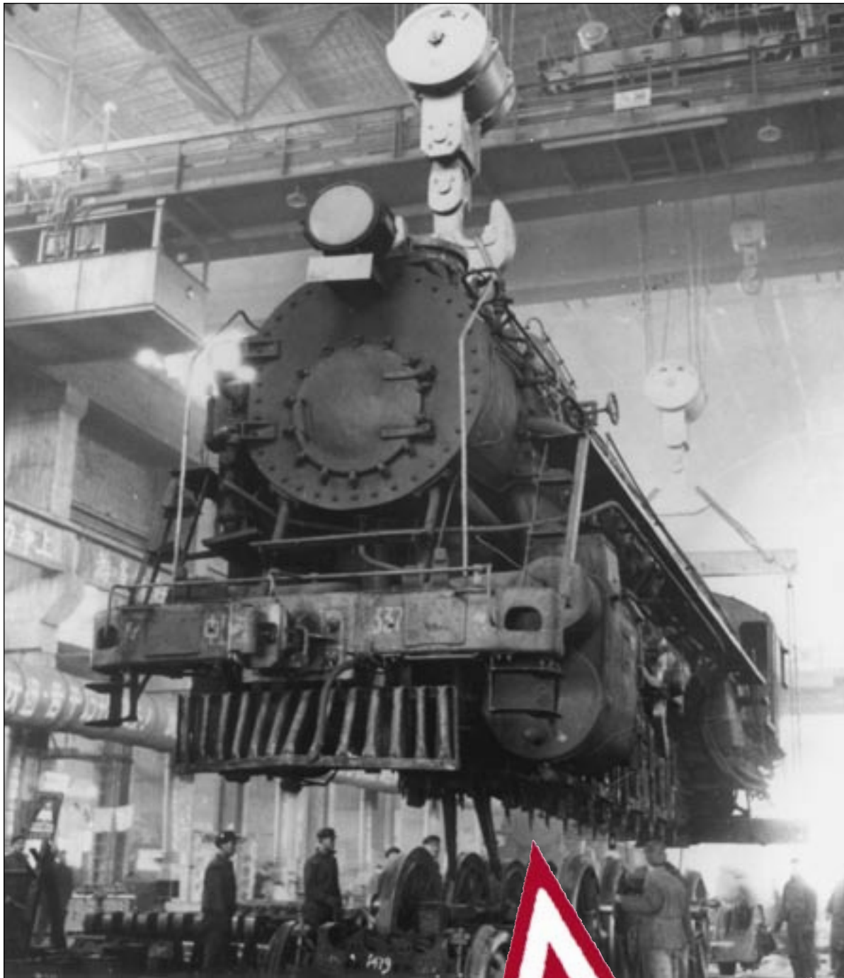
The red star was the symbol of the Soviet railways. A Russian-built 2-10-2 is being re-gauged at Changchun Works, China, around 1959.
