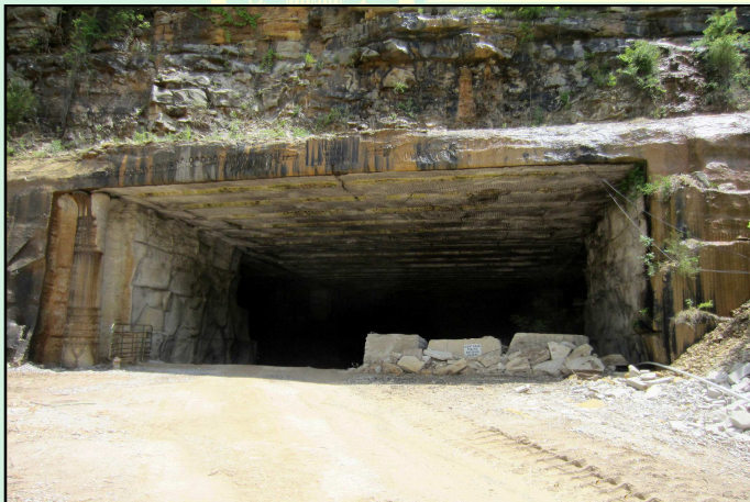
This is the second or third mine opening since the company began mining underground. The mine entrance looks to be nearly forty feet wide and about eighteen feet high. The wife of a previous owner of the company hired artisans from Russia to do the sculpturing on the left side of the entrance and across the mantle
