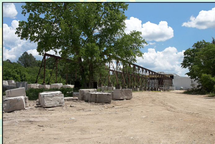
The mill building is at the far end of the gantry. Here the oolitic limestone is cut to dimension and the final finish is applied. This is the building that was converted during World War II into plant to manufacture shells for the war effort. The Fossick branch came toward the camera on the right side of the mill. There seems to be room for a small yard
