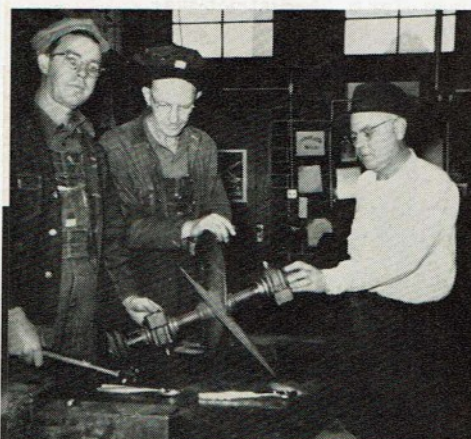
ELECTRIC SHOP , Birmingham Agency, l. to r.: Electricians J. W. Dobbs, F. L. Brockman and Foreman C. E. Lindsey. Electricians are overhauling condenser fan assembly.
