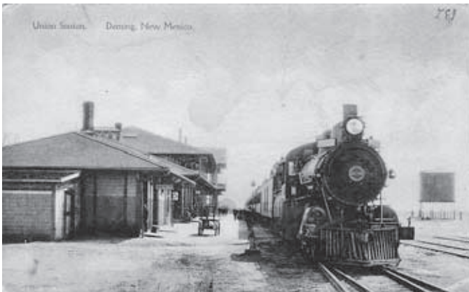
Postcard by Fred Harvey (no date) showing Southern Pacific main line train at Deming depot in its two-story form. Locomotive is SP 2280, 4-6-0 Class T-25 built by Cooke 1901.
