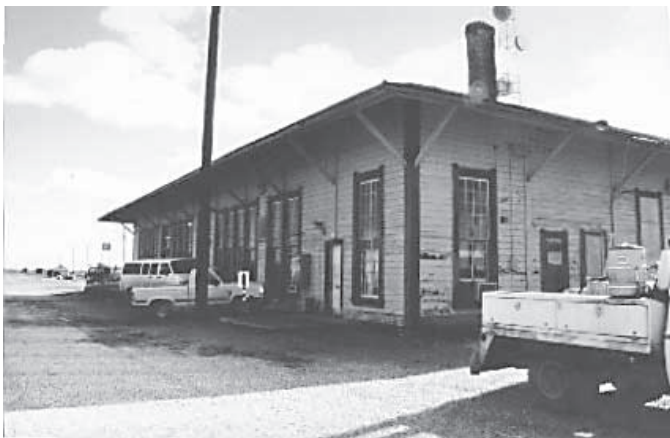
Deming depot seen from north side owned by Burlington Northern Santa Fe. Courtesy Great American Station Foundation.
