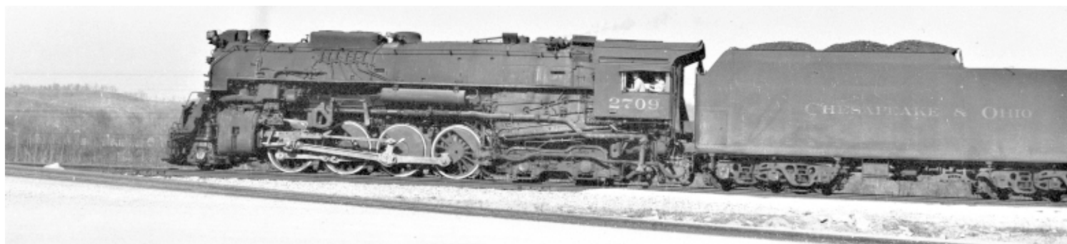
Class K-4, 2709, built by Alco in 1943, runs west along the Ohio River west of Greenup, Kentucky, in April 1953. Cab on C&O's 2-8-4 is slightly larger than on NKP's or PM's 2-8-4. Photo by E. L. Huddleston, Collection C&O Historical Society #1790.
