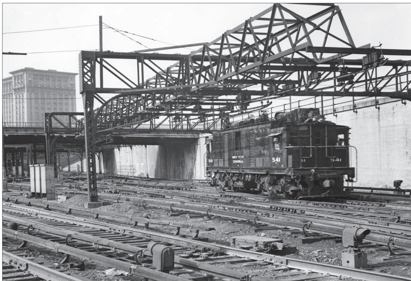
NYC 541 switching south of Detroit, Michigan's passenger station in September, 1952. A maze of slip-switches here caused extensive gaps in the third rail, requiring overhead contacts to ensure an uninterrupted power supply. Thomas Dworman photo.
