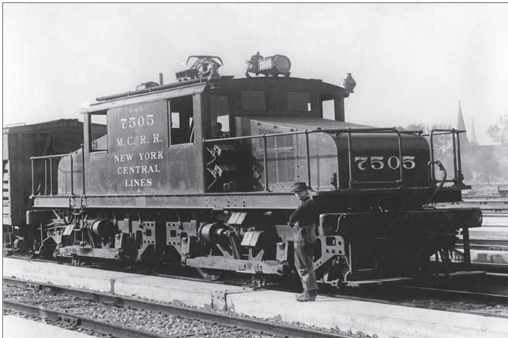
Michigan Central 7505 shows the typical mounting of a third rail shoe, as well as the miniature overhead pantograph that the New York Central used to assure uninterrupted power supply during movement through complicated track locations. Library of Congress
