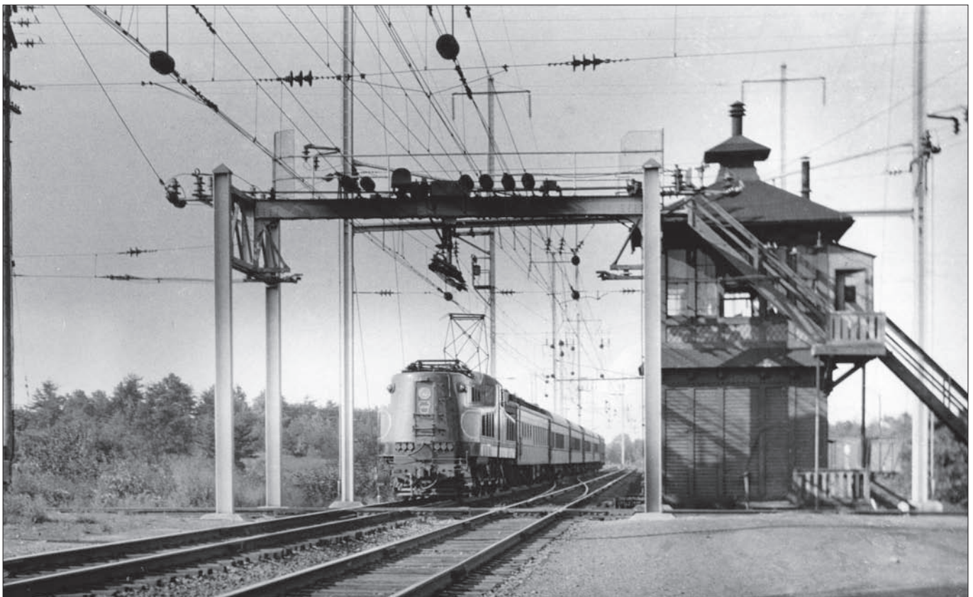
P5a on the Pennsylvania Railroad at the Washington, Baltimore & Annapolis crossing, Odenton, Maryland 1935. At this location, the PRR's 11,000 volt A.C. catenary had to cross with the WB&A's 1200 volt D.C. wire. James P. Shuman photo
