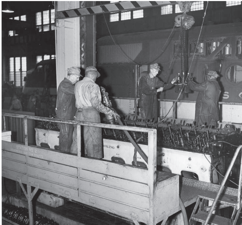
Machinists and helpers remove cam shafts and assemblies from a diesel engine in the early 1950's. SRHA Collection at the Southern Museum.
