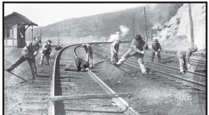
Workmen using new method of leveling tracks October 28, 1918. Penn Central Corporation Collection of Pennsylvania Railroad Negatives. Courtesy of Hagley Museum & Library, Wilmington, Delaware
